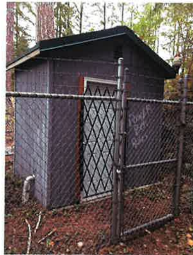
Booster Station Pump House
