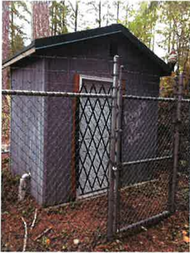
Booster Pump House
