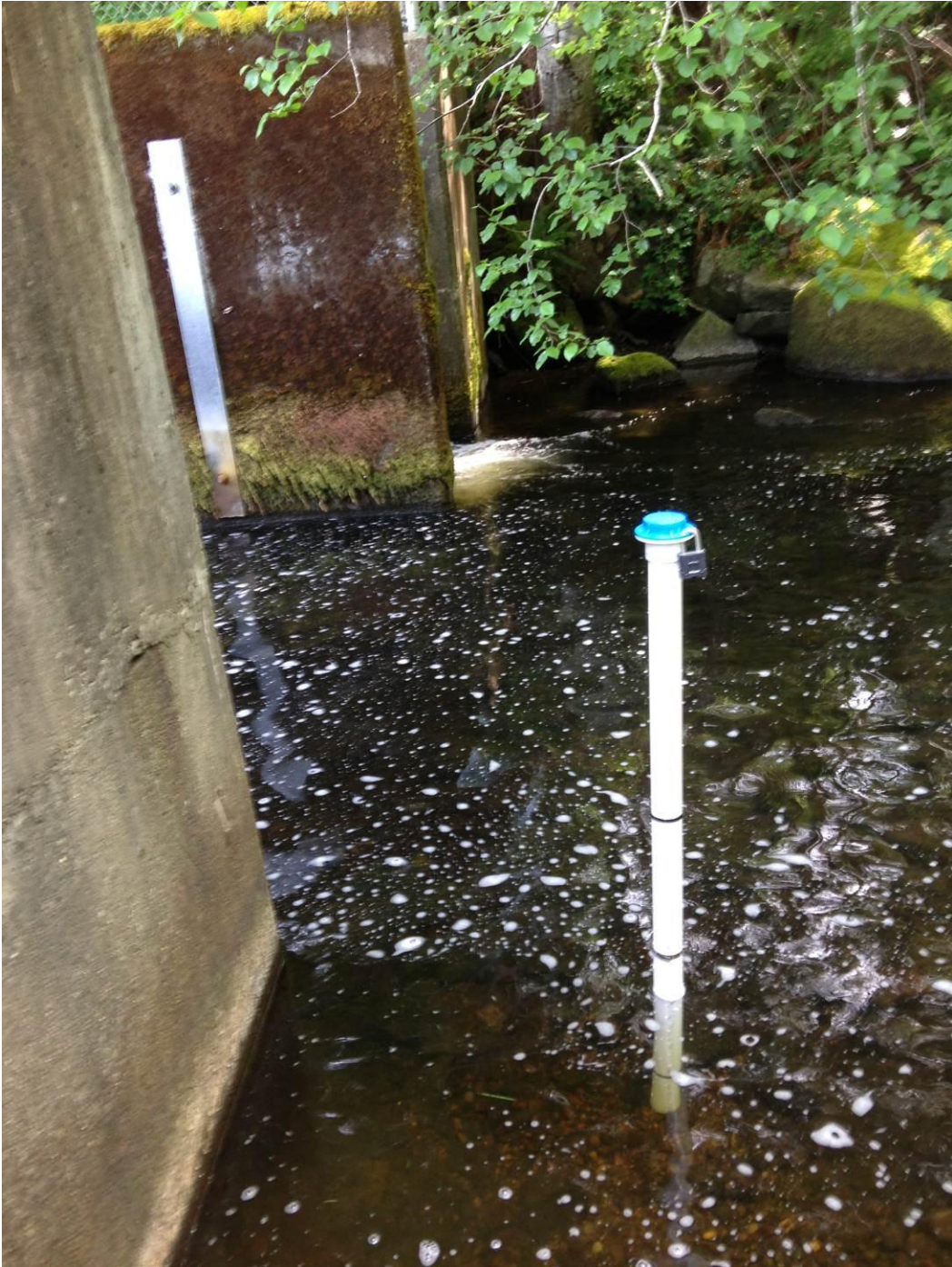
Figure 10. Level logger located below the Lake Limerick dam site.
