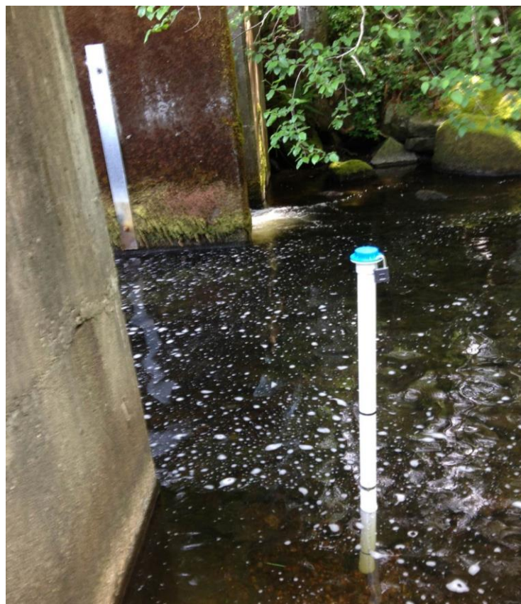
Figure 12 – Level logger located below the Lake Limerick dam
