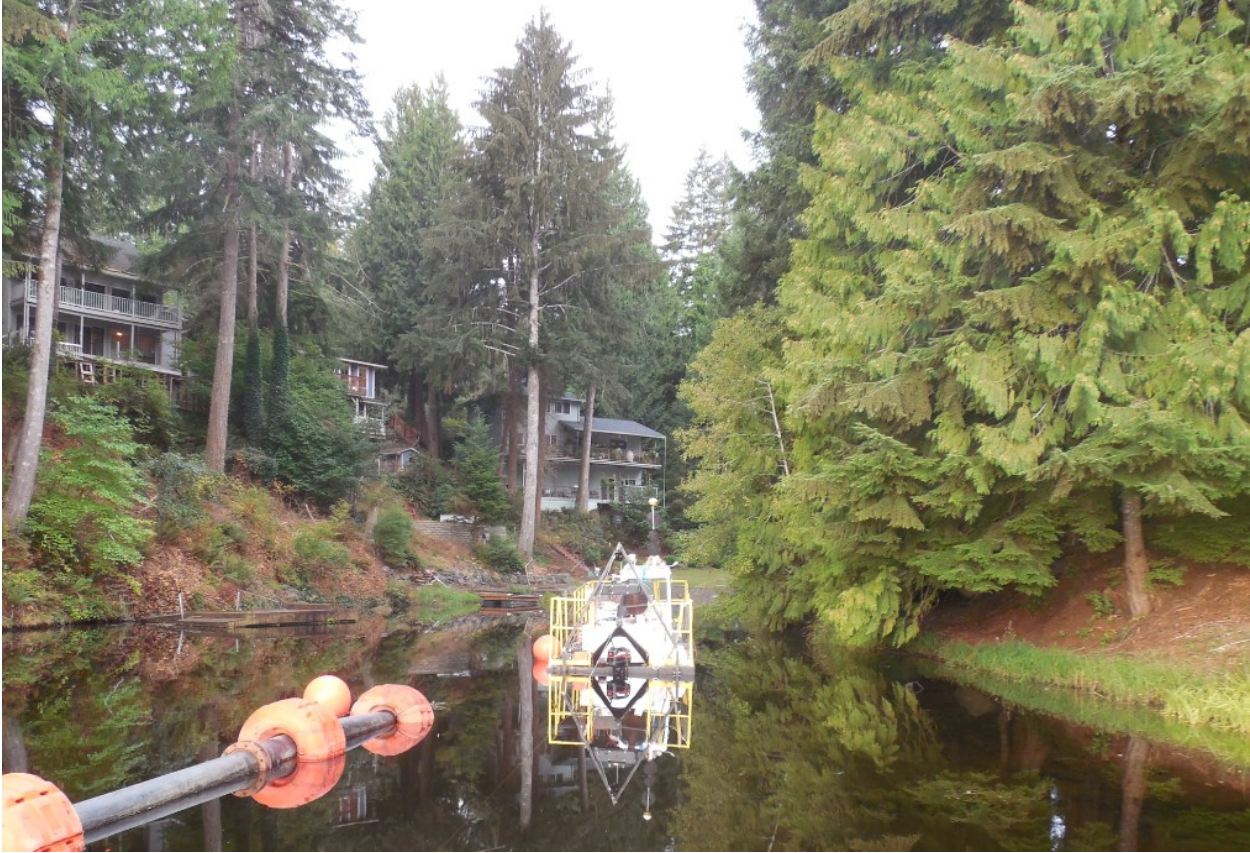
MudCat Set Up in Cranberry Creek
