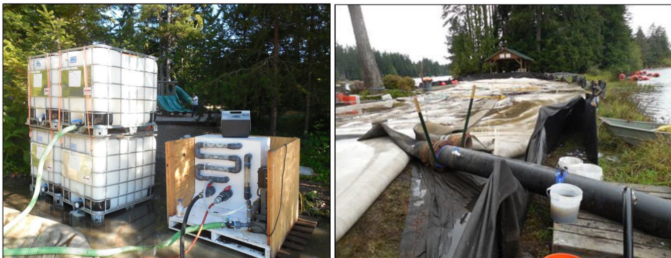
Figure 16 – Injection of flocculent into dredge material
