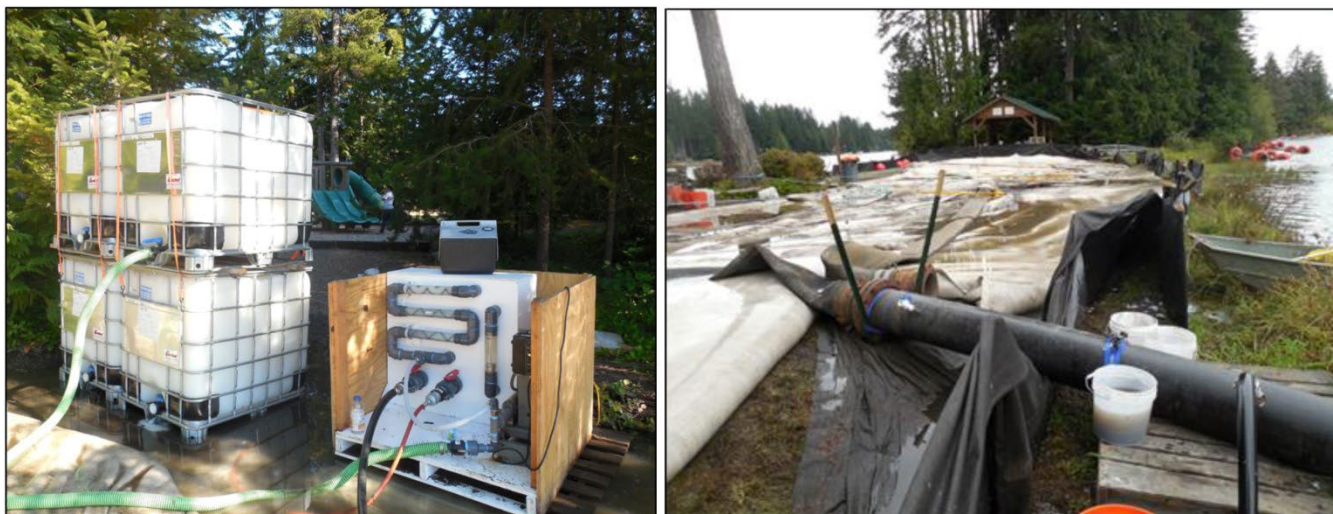
Figure 7-5– Injection of flocculent into dredge material
