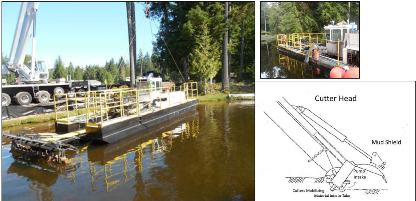
Figure 7-3 – Equipment used to conduct dredging in Lake Limerick
