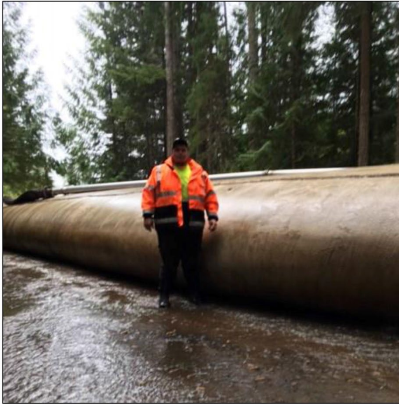
Figure 7-7 - De-watering of dredge material
