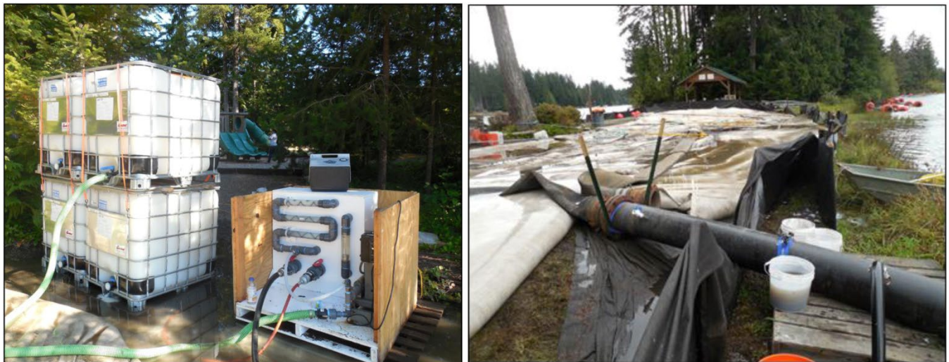
Figure 7-5– Injection of flocculent into dredge material
