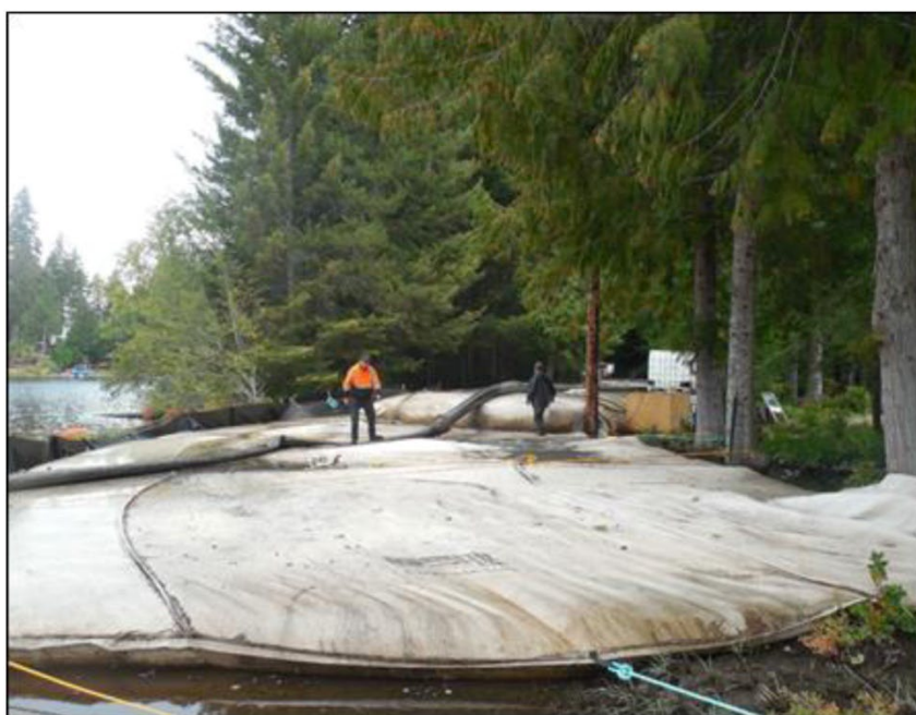
Figure A2-6. De-watering bags
