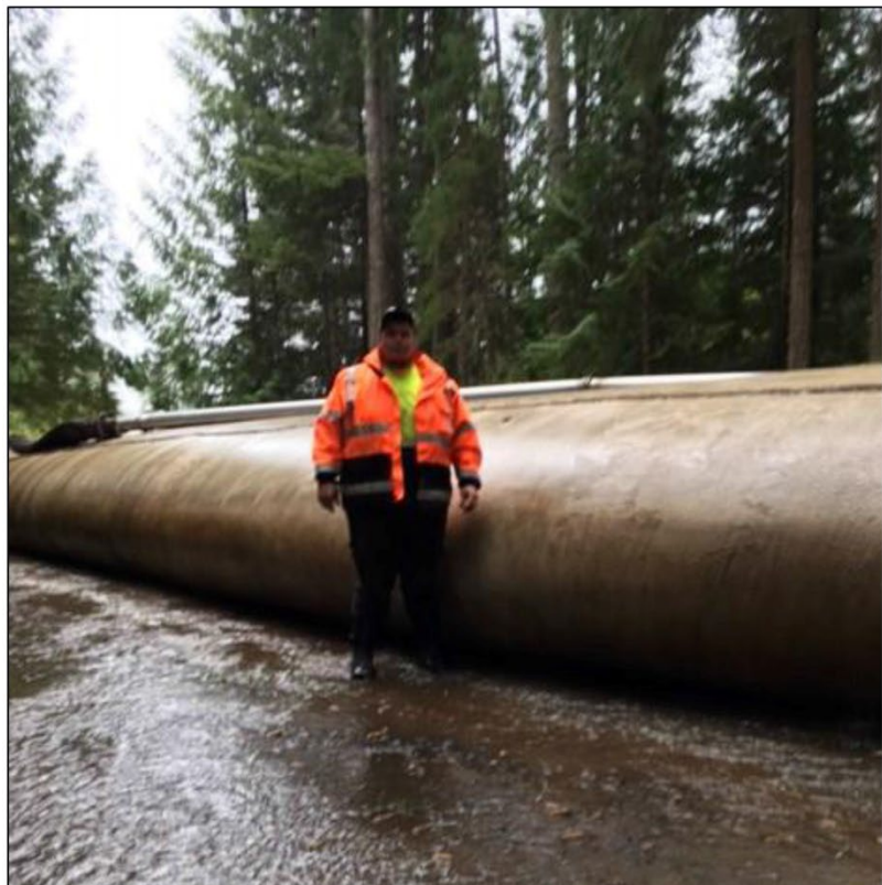
Figure A2-7. De-watering of dredge material
