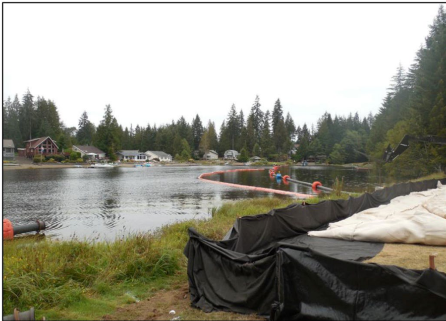
Figure A2-4. Dredging pipeline
