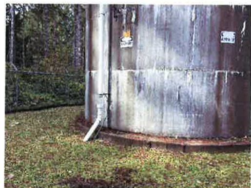
Overflow with Air Gap
