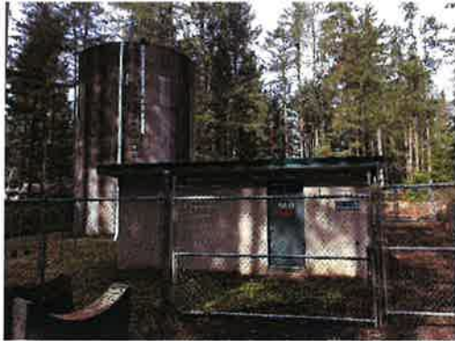
Well #4 Facilities Site
