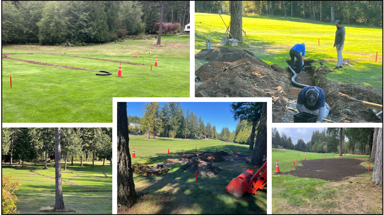
The Greens team added drainage to hole #2.
