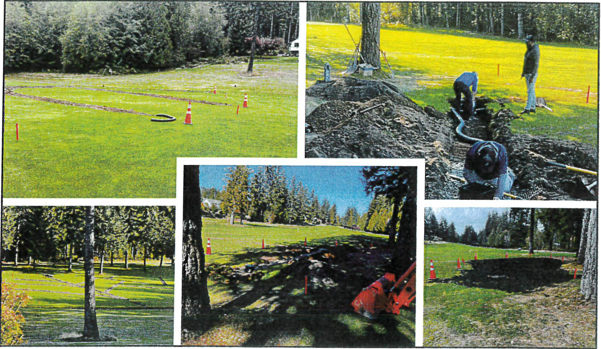
The Greens team added drainage to hole #2.
