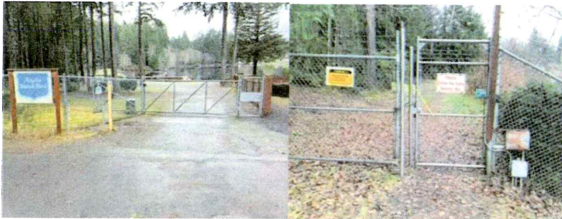
Main Entrance Gates (Anglia Park)
