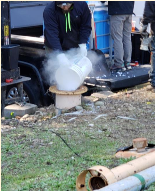
Picatti Brothers worker pours dry ice into well six to scrub the well casing to help improve capacity.
