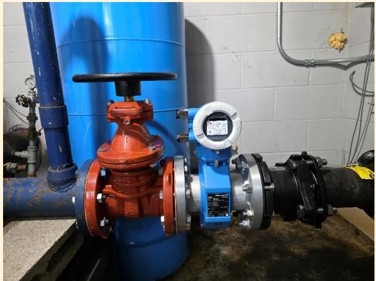
As part of the Water System Plan, new electronic source meters were installed in the spring of 2025 to replace aging mechanical meters. This will result in more precise measurement of water production. The photo shows Well #3-B.
