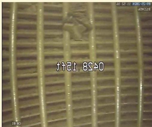
Inside Well #6 at a depth of 329 feet showing the excellent results of the dry ice scrubbing. The reversed numbers (0428.15 ft) in the center of the photo shows the total well depth.
