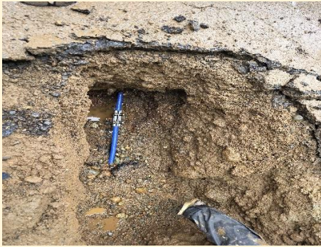
Recent water line repair on Saint Andrews Drive. We still have about 84 customers with leaks on their side of the water meter. "You fix - you SAVE!"
